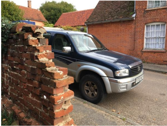
Photograph 9: Northern access view north
