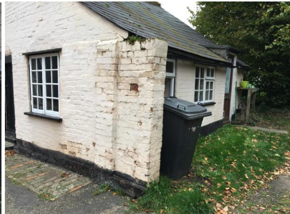
Photograph 8: Protruding wall from 1-6 The Street
